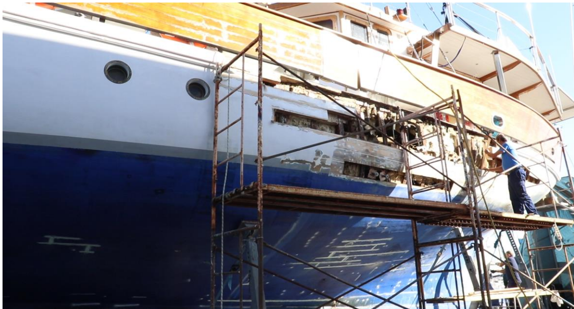
Image 1. Scaffold in a caulking operations - Source: CETEM
